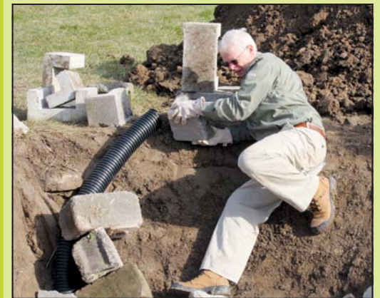
It may just look like a pit full of concrete blocks, but for a snake this could be a winter resort!
